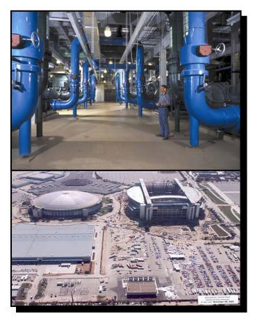
Chilled water capacity is 19,000 tons with expansion capability to 32,000 tons. Heating hot water capacity is 170 million Btuh with expansion capability to 220 million Btuh. Underground chilled and hot water distribution piping link the plant to the facilities served.
